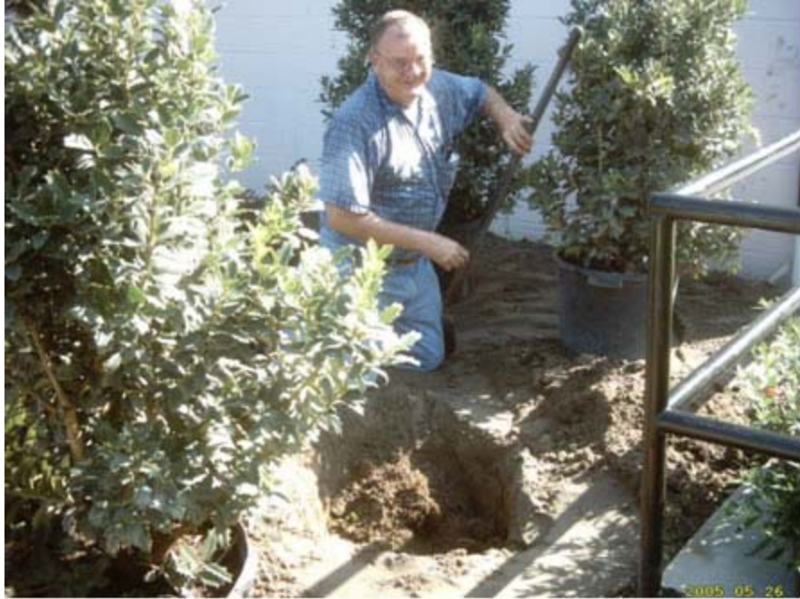
New Garden Construction
